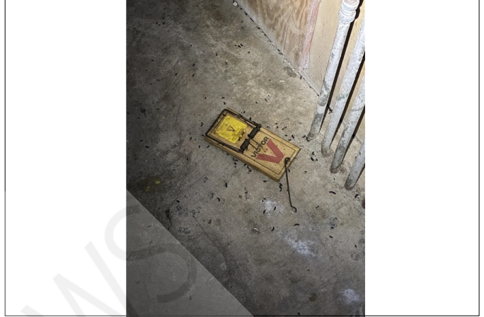
Droppings in utility closet.
